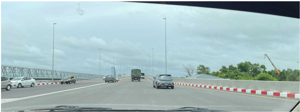
(3) Road condition of the bridge
