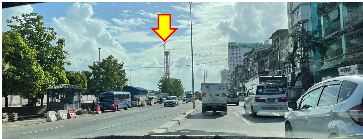
(8) Constructing condition of Friendship bridge
