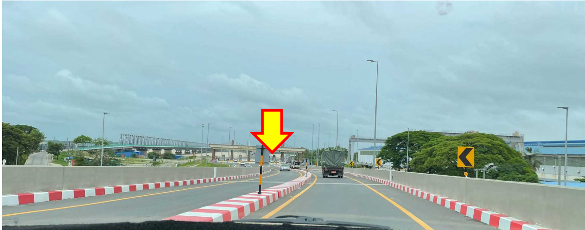
(2) Toll gate of completed bridge at Yangon side
