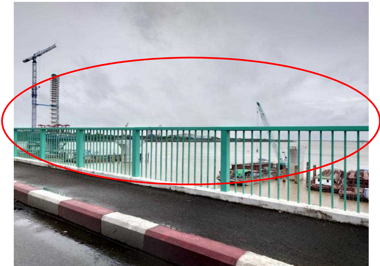
(1) Condition of the bridge in July 2023 (Under construction)
