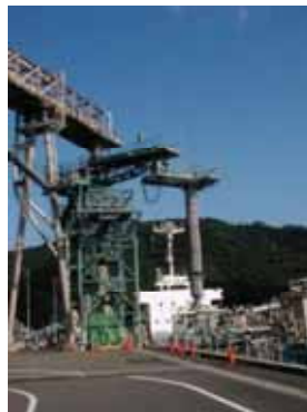
Pneumatic handling (dry process)
